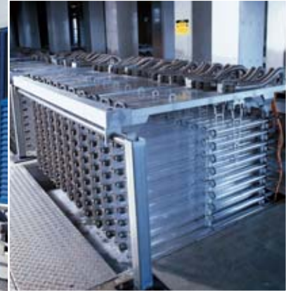
UV modules in maintenance position
