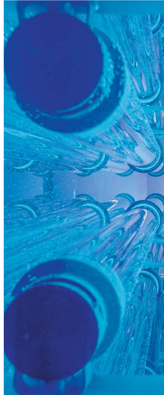
WEDECO TAK 55 UV modules in the water
