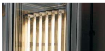
FIT D - light tubes installed in door
